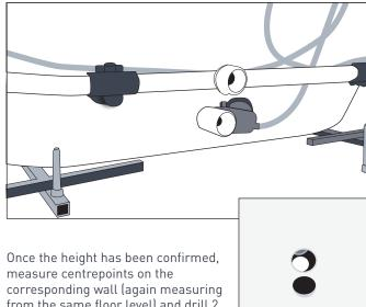
measure centrepoints on the corresponding wall (again measuring from the same floor level) and drill 2 x 75mm (minimum) holes through the wall to the exterior, or the location where the pump will be located.
